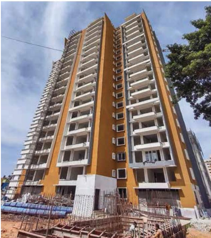
▲ Developers insist that workers adhere to safety norms.
