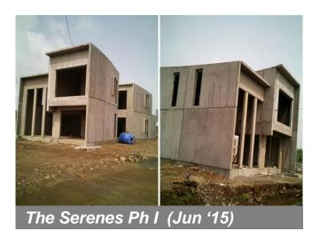
Note: Units constructed using precast technology
